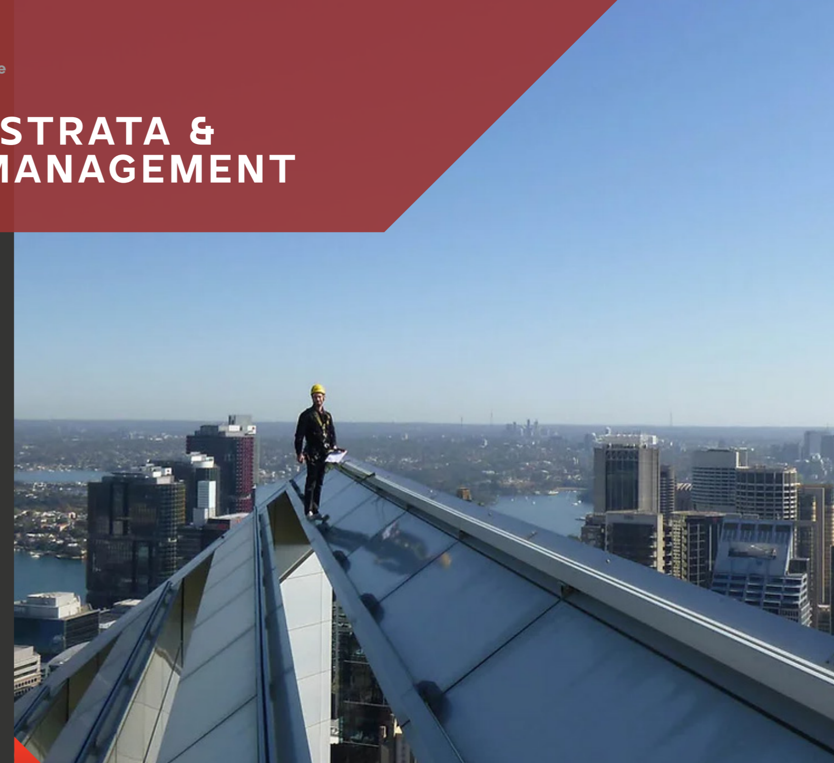
ANZ Building Roof Inspection, NSW
