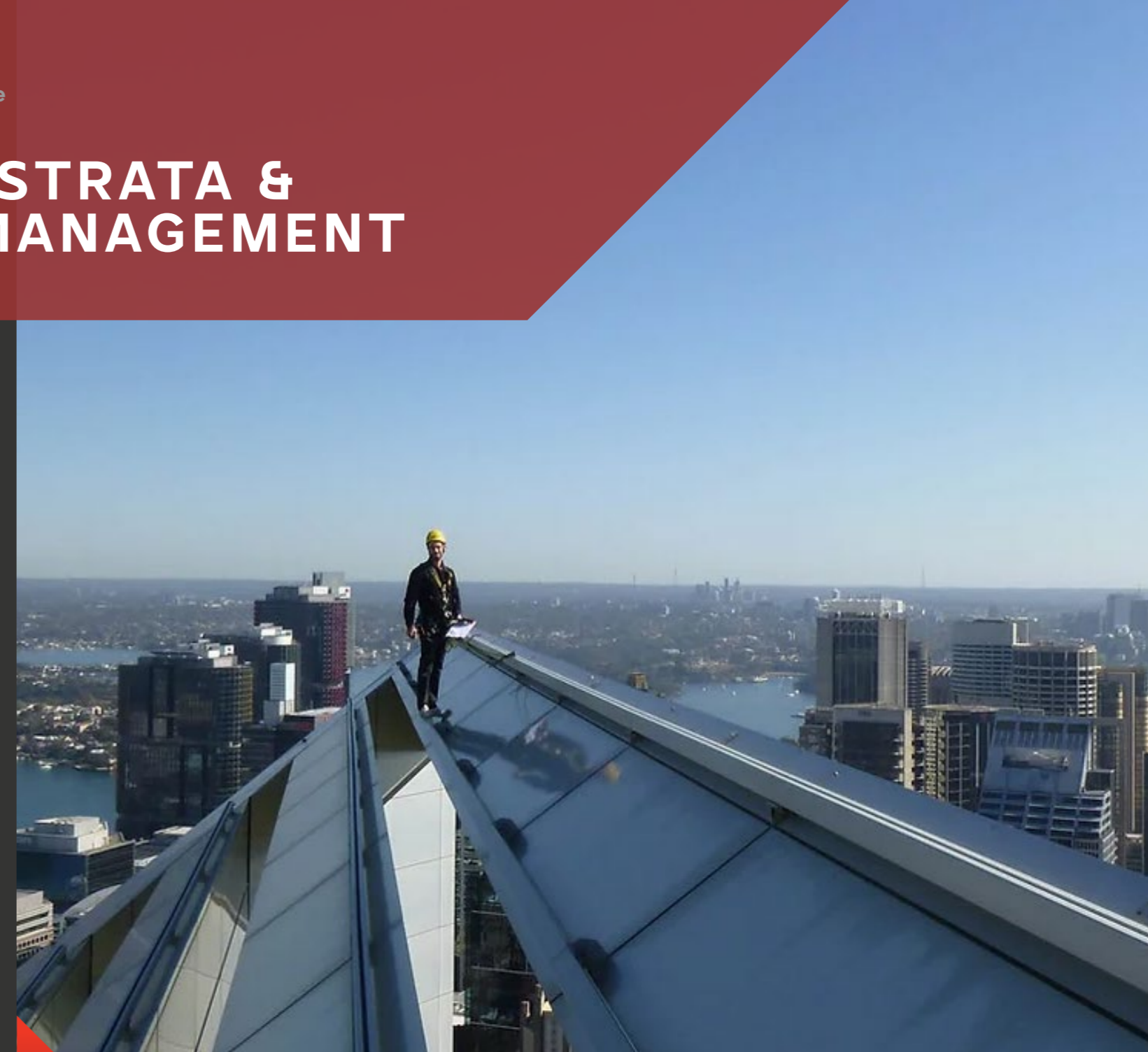
ANZ Building Roof Inspection, NSW
